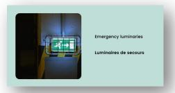
Another important issue for buildings' security is the installation of emergency luminaries Luminaires de secours. Either a conventional or an addressable luminaries control panel can be installed.
