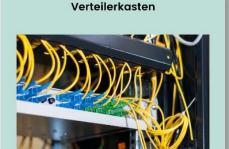
Cables with flexible copper cores are used for connecting movable devices or as individual cores in a distribution cabinet: Verteilerkasten.
