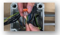
Connection terminals - colloquially known as Wago terminals. There are special connecting terminals for flexible copper wires: Federkraftklemme.
