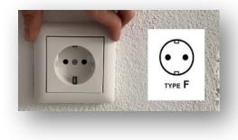
In Germany, type F sockets are used. In German socket is called: Steckdose.
