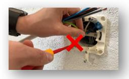
Flexible copper cores must NOT be connected directly to the screw connections of the Schuko plug.
