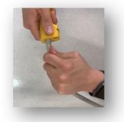
Remove the sheath insulation of the cable without damaging the insulation of the cores. For short pieces, a stripper is sufficient: Entmanteler.
